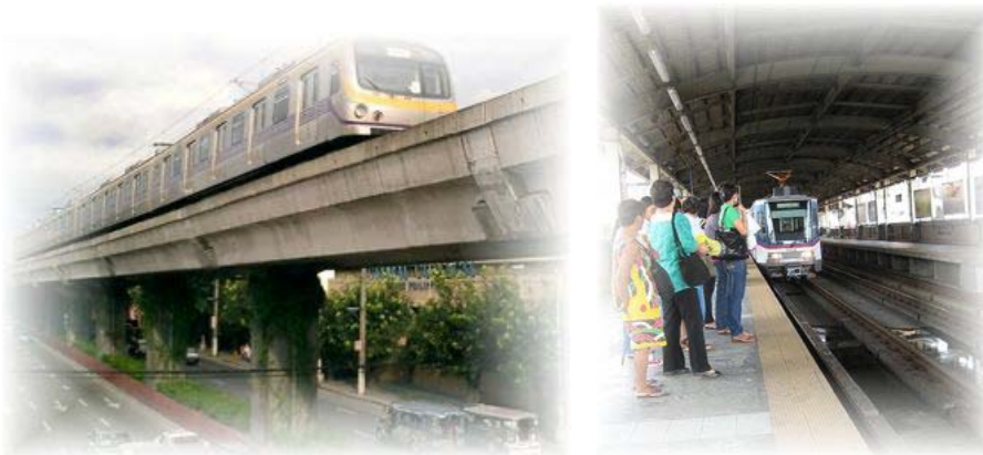
Manila - LRT on left and MRT on right
